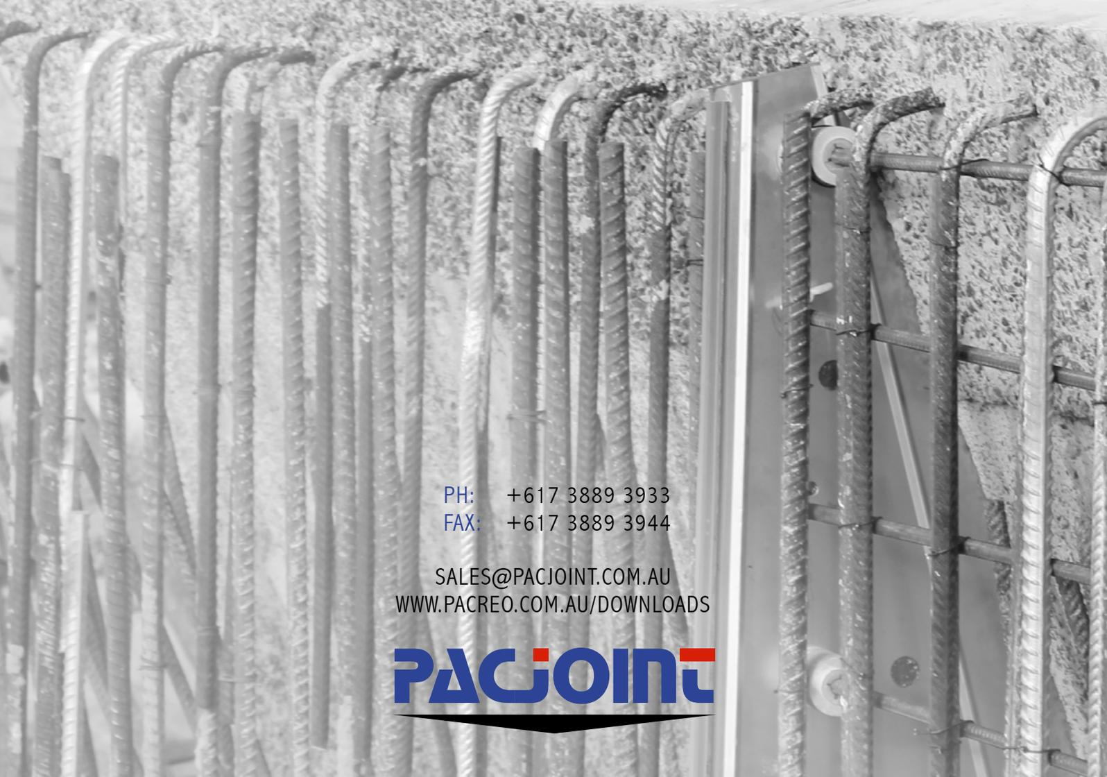
A black and white photograph of a reinforced concrete wall under construction. The wall is composed of numerous vertical rebar rods protruding from a concrete surface. To the right, a vertical metal formwork panel is visible, secured with horizontal bolts and nuts. The rebar rods are arranged in a regular grid pattern, and some have hooks at their top ends. The concrete surface is rough and textured.
